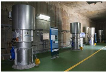
consists of 16 turbines, 18.5kW each, with an estimated overall power of 296kW. The plant started operations in July 2011.
